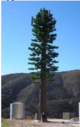
Monopine Stealth Tower
