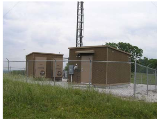
typical co-location tower site
