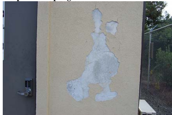
Lead paint sampling
