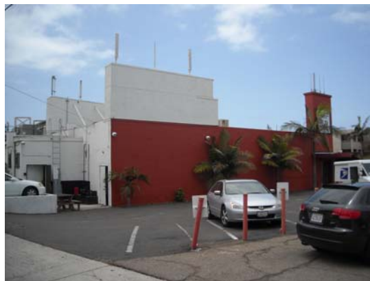
Rooftop antenna co-location
