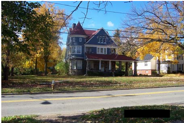
Typical Historical Structure
