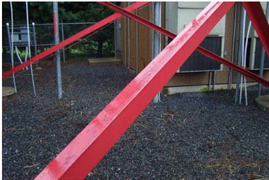
Lead Paint Sampling
